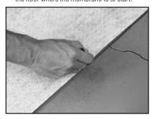
1.4 Set aside precut sections (or entire rolls) of *Mapeguard 2*. Continue with installation instructions at Step 2.3.
